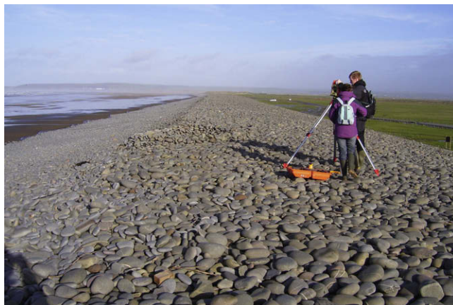
Fig. 6. Westward Ho! Devon, where a large wave caused damage and injury to bathers on 31st July 1966 (photo taken January 2007; view towards the north).
